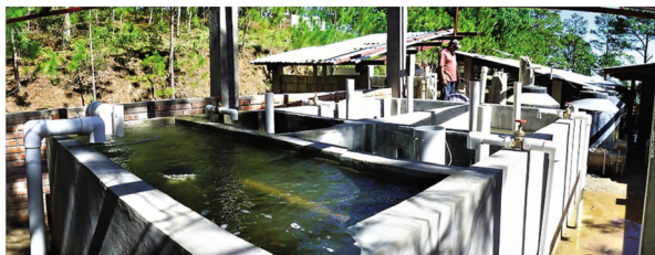
FIGURE 5.3 Grit chamber in Honduras.
